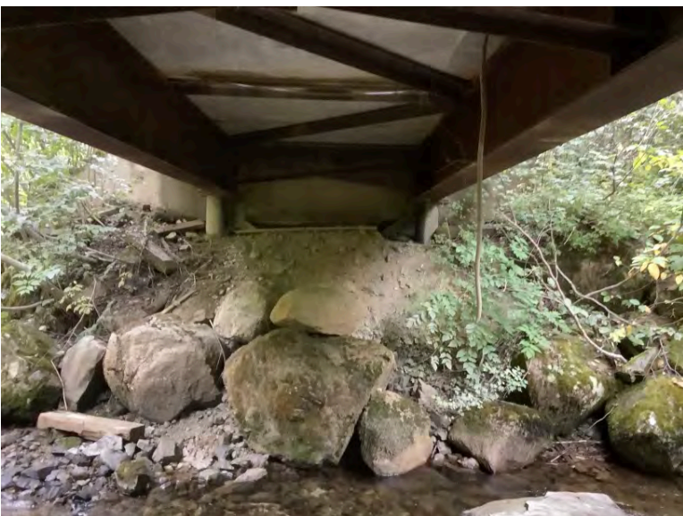
Right Bank Abutment when facing downstream
