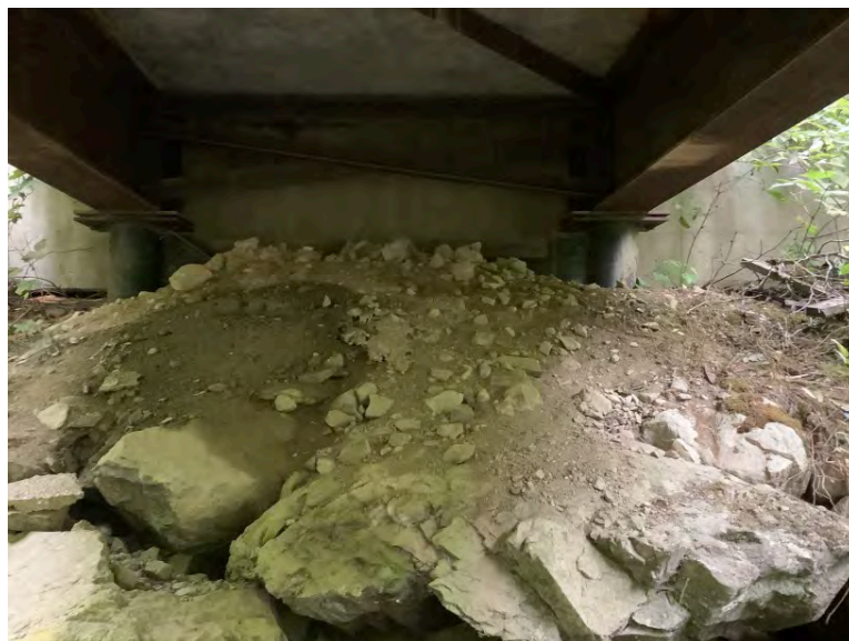
Left Bank Abutment when facing downstream
